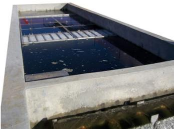
The COS Series, Concrete Coalescing Oil Water Separators are designed for applications where a high performance coalescing separator design is desired using Flopak coalescing media. The industrial duty COS design offers many features such as solids V-hopper, sludge auger, adjustable water weir, integral inlet diffuser, and many options to provide engineers, system integrators and end users with convenience and flexibility in oil separator system configuration choices.
