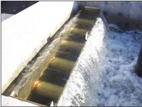
Concrete API-CPI 6,000 GPM
