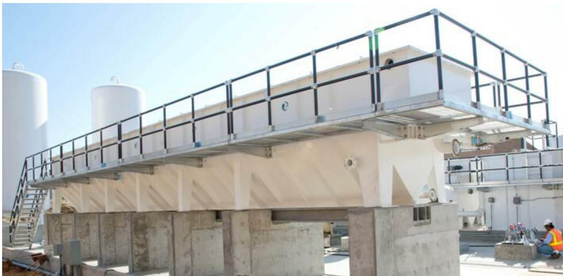
Elevated API combined with CRT chemical treatment system and DAF
